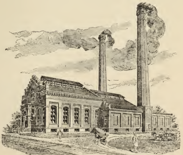
PUMPING STATION, ARTESIAN WATER WORKS.
